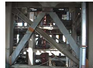
Fig.8 Cross Brace Damper
